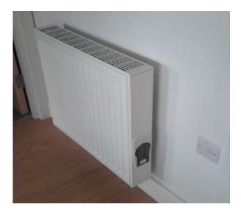
The above image shows one of the apartment radiators and its fuse spur on the wall to the right. Under the grey panel on the side is a round white switch. Turning the switch increases or decreases the heat output of that individual heater.
